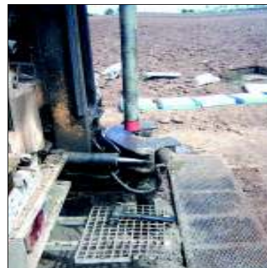
Picture 4: Detail of the drill string
