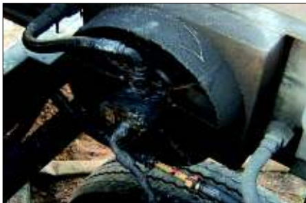
Photo 2: Leakage sleeve with cooling fan detail
