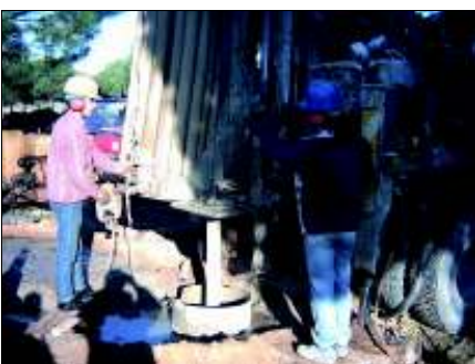
Photo 4: View of drilling workers.
