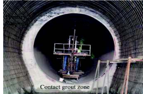
Figure 2. Contact grout between pipe and support
