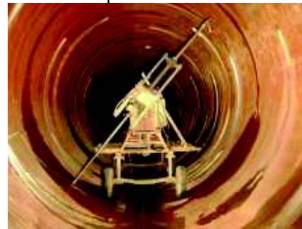
Figure 3. SMS rotary type drilling machine
