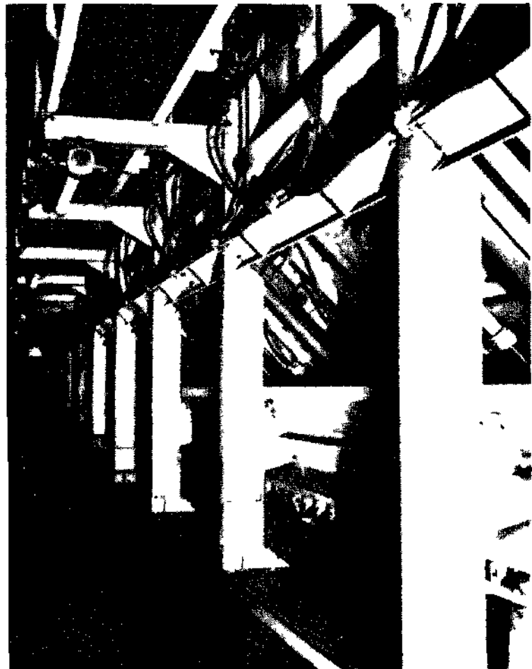
Figure 12a. Underground installation of 900 tonne static bunker (Kellingley Colliery).
