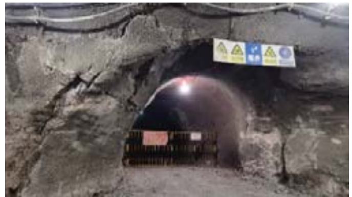
Fig.1 Ore pass door in the mining area
